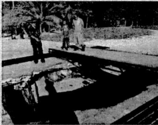
Jun Sablan and two boys stand next to the damaged portion of Sugar Dock.
